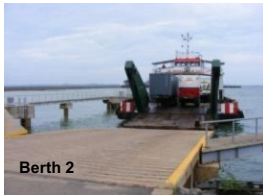
Berth 2 ( roro ramp ) - for RoRo operation with Landing Craft /LCT, water draft up to 5m LWS
