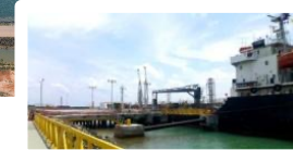
Berth 4 ( liquid jetty ) - for liquid cargo
